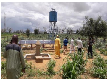
Provisional drilling for water access
